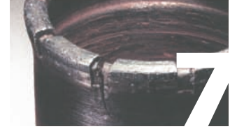
CRACKS IN THE WATER WAYS
